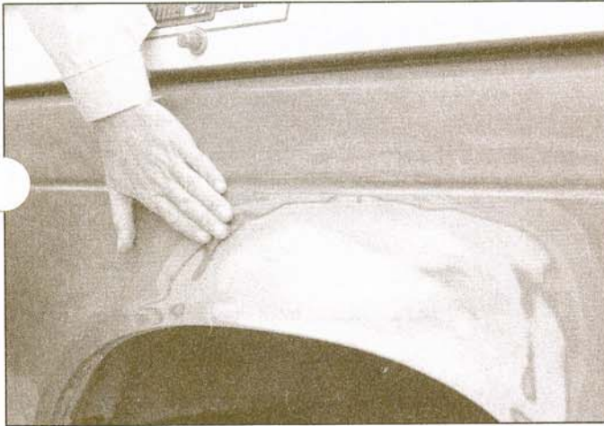
9 You shouldn't be able to feel any ridge at the transition from the filler to the bare metal or from the bare metal to the old paint. As soon as the repair is flat and uniform, remove the dust and mask off the adjacent panels or trim pieces
