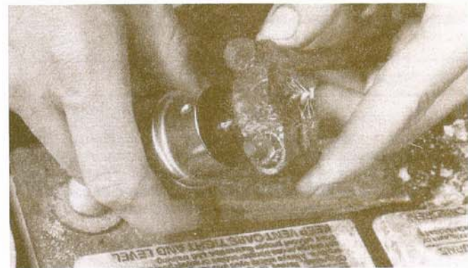
8.7b When cleaning the cable clamps, all corrosion must be removed (the inside of the clamp is tapered to match the taper on the post, so don't remove too much material)
